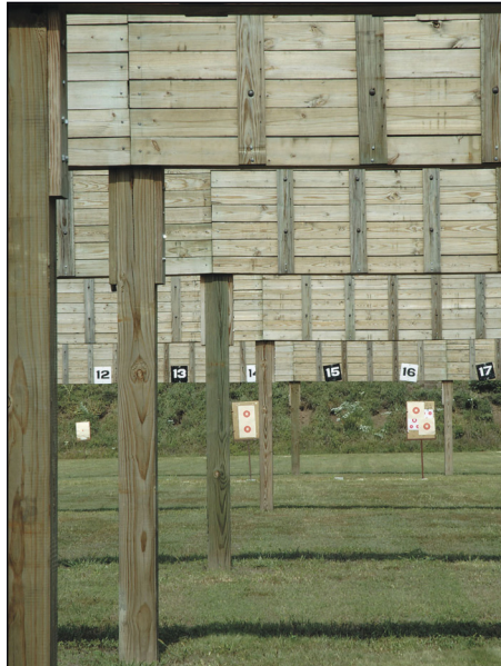
Baffles in place at the Fancy Creek Range ensure no rounds leave the range.
